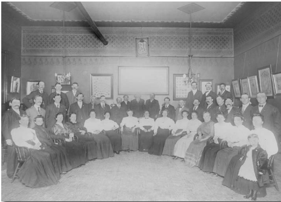
This uncaptioned photo was found in a cabinet and may date before the third level addition of 1918. It will be a historical reference and visual document for our building and perhaps for any restorative work in the future.
