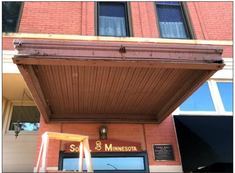
C.S.P.S. Hall Michigan Street Canopy
